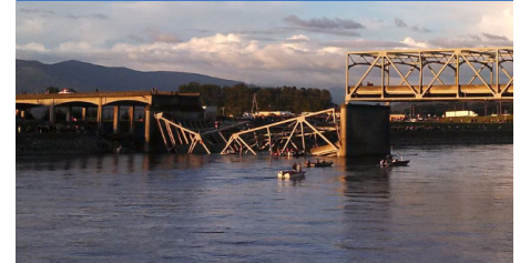
The I-5 Skagit River bridge collapsed in 2013 in part due to its obsolete design
